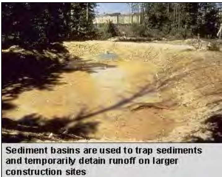
FIGURE 5-9 Sediment basin. SOURCE: EPA NPDES Menu of BMPs (available at http://cfpub.epa.gov/npdes/stormwater/menuofbmps/index.cfm?action=factsheet_results&view=specific&bmp=56 ).
