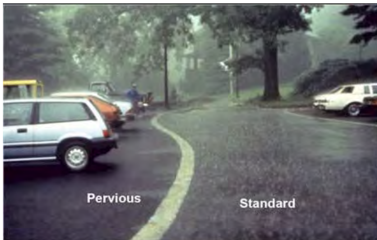
FIGURE 5-29 Porous asphalt. SOURCE: PaDEP (2006).
