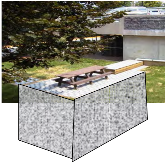
FIGURE 5-30 A retrofitted infiltration trench at Villanova University. SOURCE: Reprinted, with permission, from VUSP. Copyright by VUSP.
