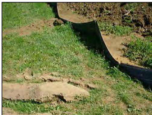
FIGURE 5-7 A functioning silt fence (top) and an improperly maintained silt fence (bottom). SOURCES: Top, EPA NPDES Menu of BMPs (available at http://cfpub.epa.gov/npdes/stormwater/menuofbmps/index.cfm?action=factsheet_results&view=specific&bmp=56 ) and, bottom, Robert Traver, Villanova University.
