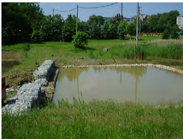
FIGURE 5-44 Villanova University sediment forebay. SOURCE: Reprinted, with permission, from VUSP. Copyright by VUSP.
