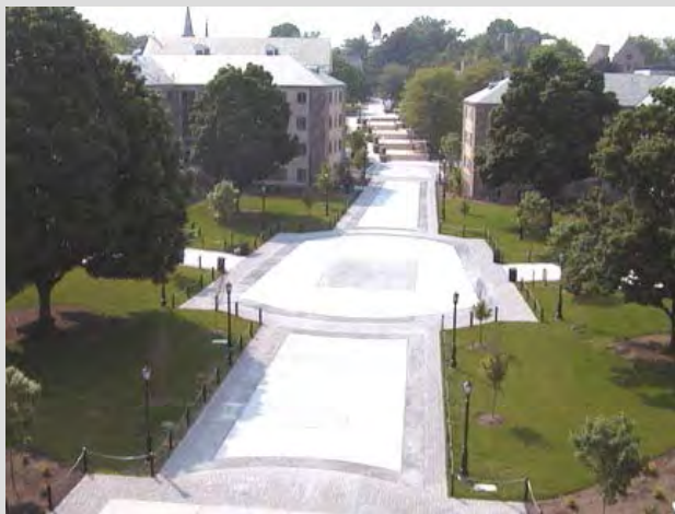
FIGURE 5-33 Villanova University pervious concrete retrofit site. SOURCE: Reprinted, with permission, from VUSP. Copyright by VUSP.
