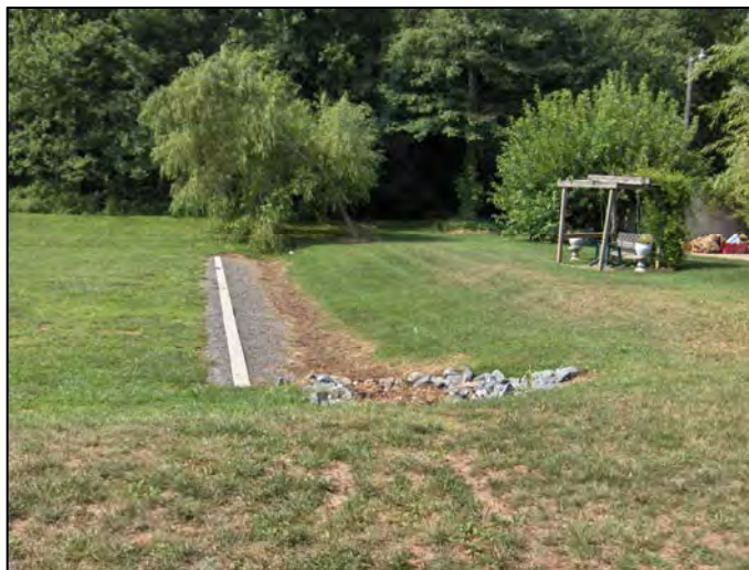
FIGURE 5-11 Level spreader. SOURCE: Robert Traver, Villanova University.
