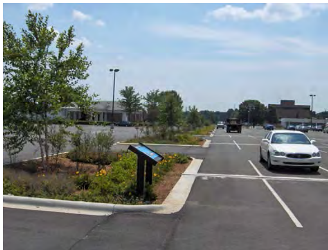
FIGURE 5-27 North Carolina Retrofit Bioretention SCMs. SOURCE: Robert Traver, Villanova University.
