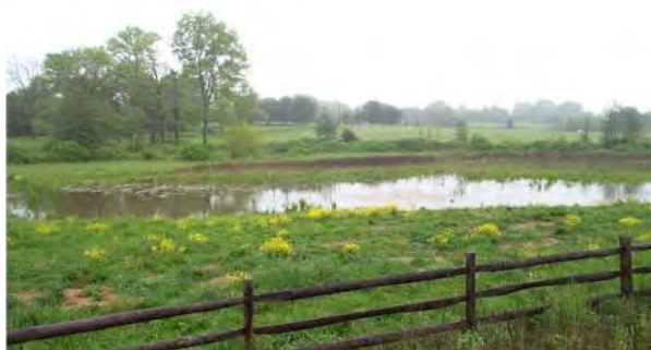
FIGURE 5-42 Wet pond. SOURCE: PaDEP (2006).
