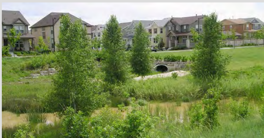
FIGURE 5-56 A consolidated treatment area adjacent to one of several neighborhoods that have been constructed as part of the project's build-out. SOURCE: Courtesy of Wenk Associates.
