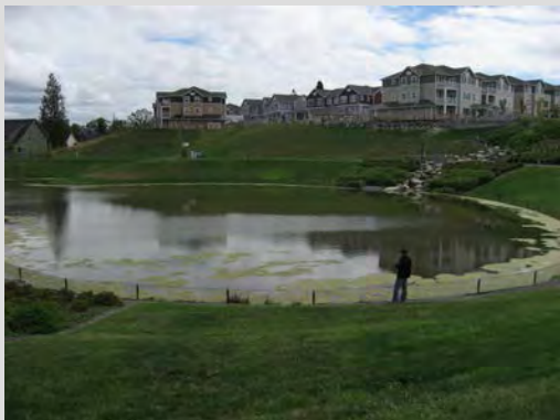
FIGURE 5-58 Natural drainage system methods have been applied to a 34-block, 1,600-unit mixed-income housing redevelopment project called High Point. Shown on top, vegetated swales, porous concrete sidewalks, and frontyard rain gardens convey and treat stormwater on-site. Below is the detention pond for the development. SOURCE: top, William Wenk, Wenk Associates, and bottom, Laura Ehlers, National Research Council.
