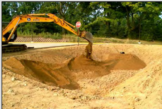
FIGURE 5-22 Placement of the mixed soil in the basin. Notice the construction equipment being kept away from the basin to avoid potential compaction of the sub-base. SOURCE: Reprinted, with permission, from VUSP. Copyright by Villanova Urban Stormwater Partnership.
