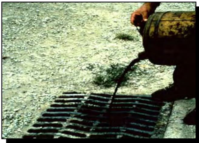
FIGURE 3-29 Contamination of storm drainage with inappropriate disposal of oil. SOURCE: Courtesy of the Center for Watershed Protection.
