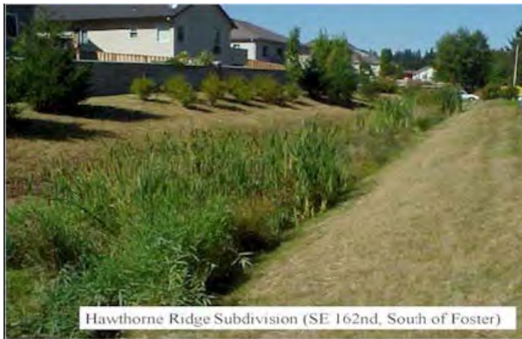
FIGURE 5-16 Vegetated swale. SOURCE: PaDEP (2006).
