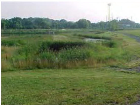
FIGURE 5-40 Constructed wetland. SOURCE: PaDEP (2006).
