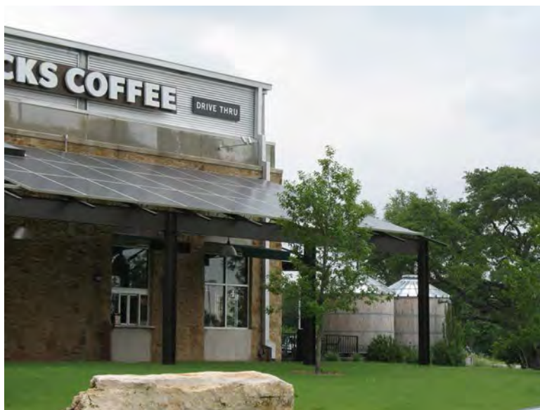
FIGURE 5-14 Rainwater harvesting tanks at a Starbucks in Austin, Texas. SOURCE: Laura Ehlers, National Research Council.
