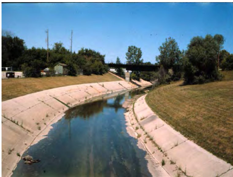
FIGURE 5-2 Concrete channel in Lincoln Creek, Milwaukee, Wisconsin. SOURCE: Roger Bannerman, Wisconsin Department of Natural Resources.
