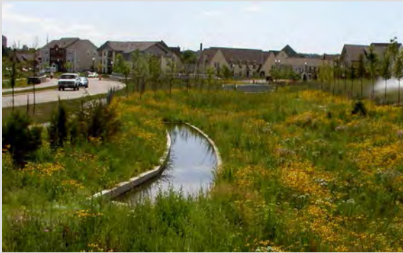
FIGURE 5-57 View of a sediment trap and porous landscape detention area in the central parkway spine of Heritage Park. The sediment trap in the center left of the photo was designed for ease of maintenance access by city crews with standard city maintenance equipment. SOURCE: Courtesy of the SRF Consulting Group, Inc.
