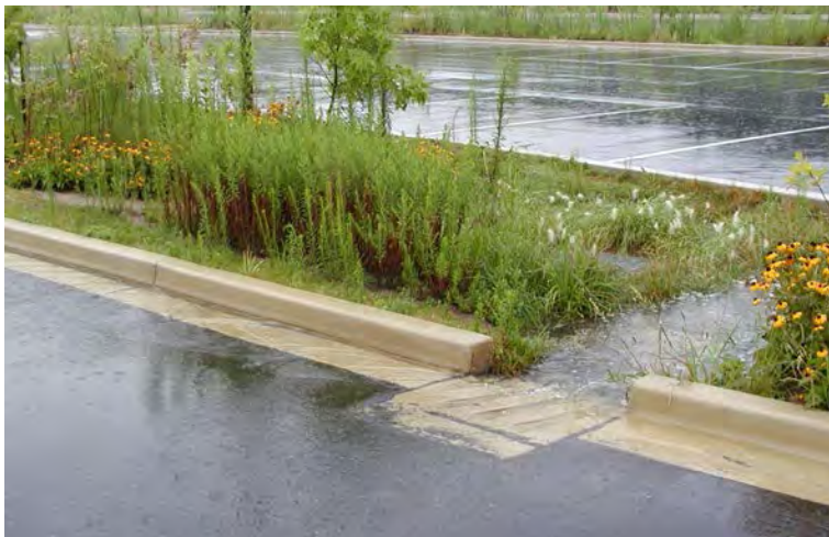
FIGURE 5-17 Bioretention during a storm event at the University of Maryland. SOURCE: Reprinted, with permission, from Davis et al. (2008). Copyright 2008 by the American Society of Civil Engineers.
