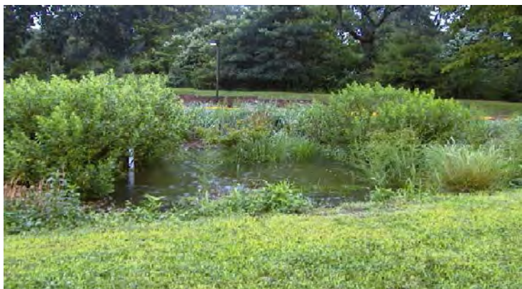
FIGURE 5-19 Retrofit bioinfiltration at Villanova University immediately following a storm event. SOURCE: Robert Traver, Villanova University.
