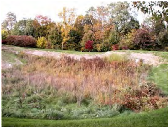
FIGURE 5-43 Dry extended detention pond. SOURCE: PaDEP (2006).
