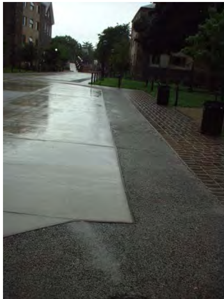
FIGURE 5-31 Pervious concrete at Villanova University. SOURCE: Reprinted, with permission from Villanova University. Copyright by VUSP.
