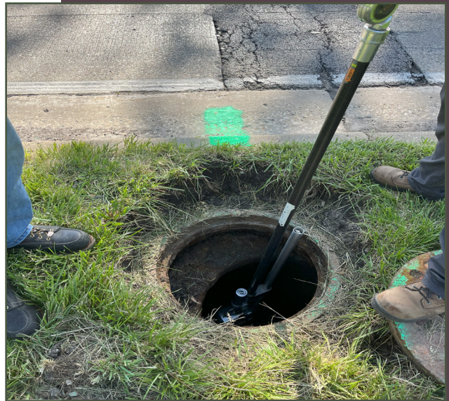
Lake County Public Works deploying a pole camera in a manhole (activities performed in the Des Plaines River watershed).
